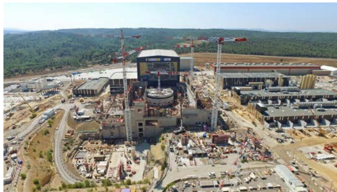
The Tokamak building under construction
