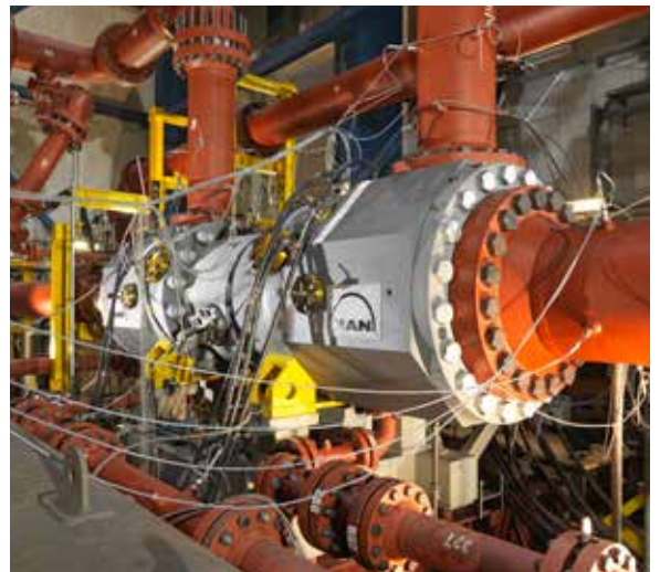
Shop test of a MOPICO® unit
